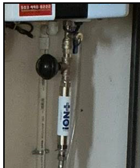
HALO unit installed on a tankless water heater
